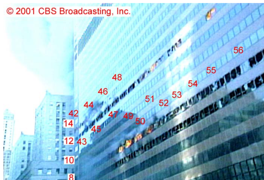
Figure 5–134. View of the north face of WTC 7 taken from a video recorded from inside the lobby of 123 Barclay Street at 3:44 p.m. ± 4 min.
