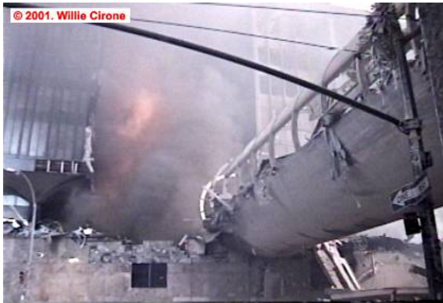
Figure 5–19. Image of the Pedestrian Bridge taken from a video shot shortly after the collapse of WTC 1 from near the corner of West Broadway and Vesey Street. The buildings across Vesey Street are WTC 5 (left) and WTC 6 (right). The image intensity has been adjusted.
