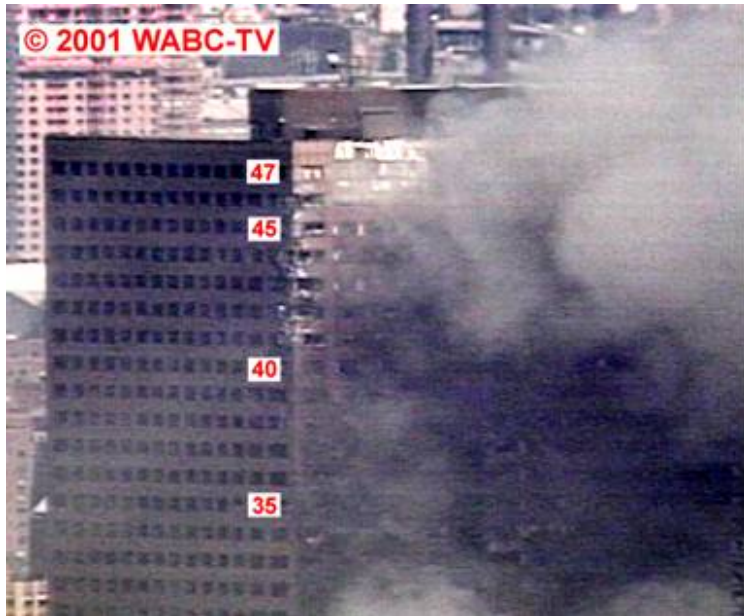
Figure 5–80. Cropped view of the south face of WTC 7 taken from a video shot from a helicopter hovering to the southwest of the WTC site around 1:00 p.m. The intensity levels have been adjusted, and floor numbers have been added.
