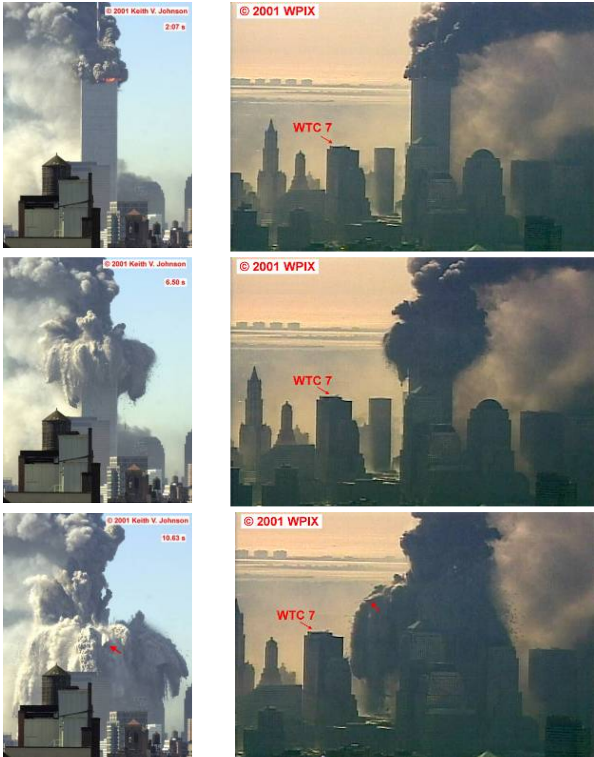
Figure 5–40. A series of cropped photographs shot from the north and frames from a video shot from the west show the collapse of WTC 1.
