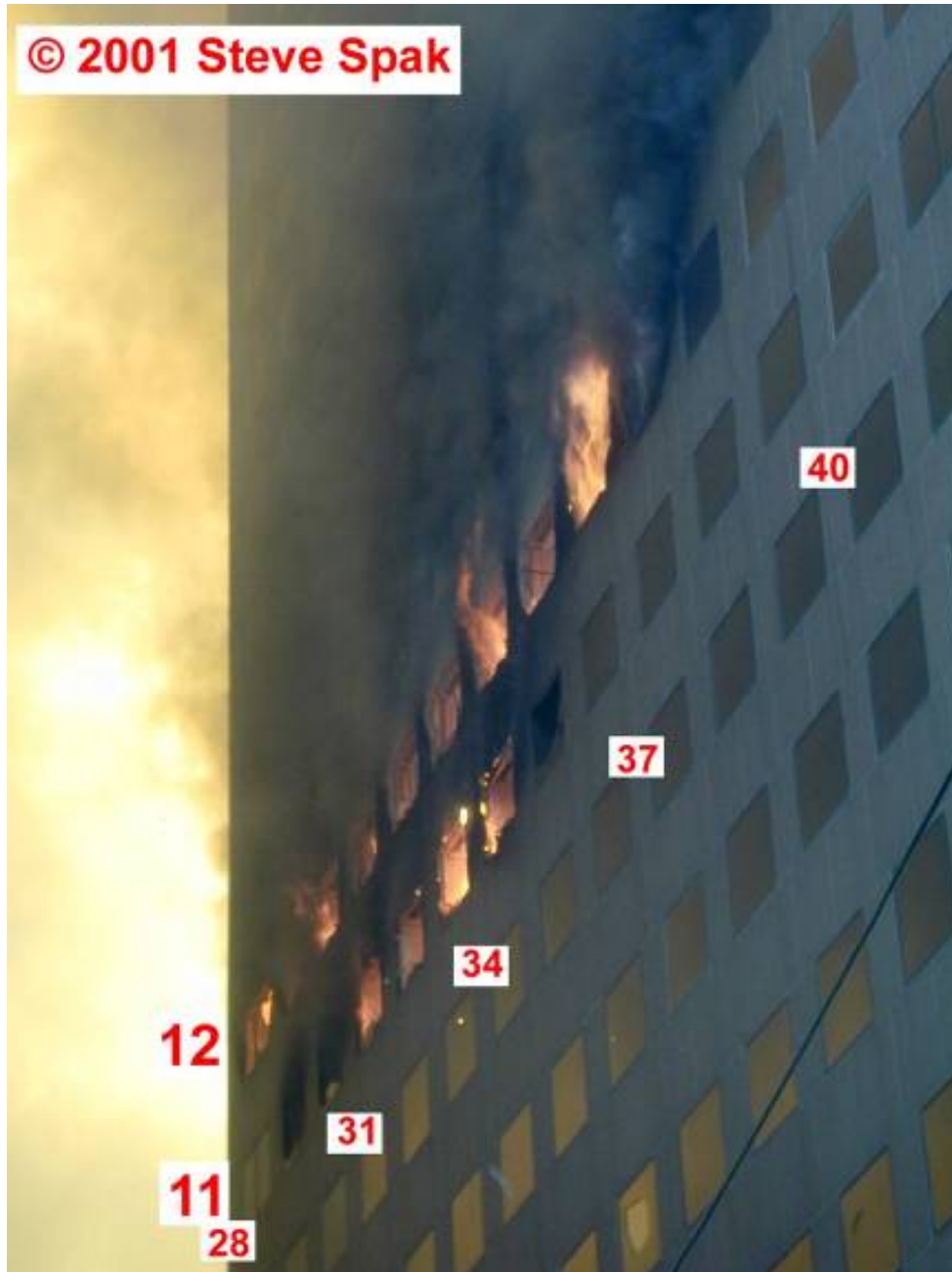
Figure 5–117. Photograph showing fires on the east face of WTC 7 at 2:28:43 p.m. ± 1 s. The intensity levels have been adjusted, and column and floor numbers have been added.
