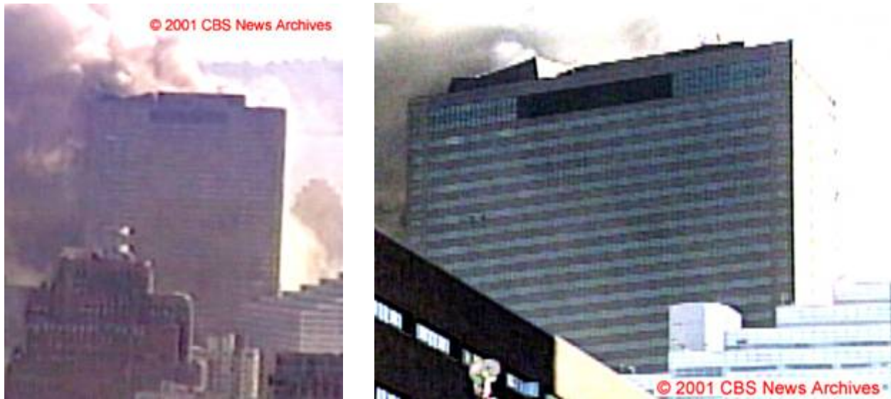
Figure 5–193. Cropped frames from the Camera 2 video clip and the Camera 3 video clip, showing the north face of WTC 7 1.0 \text{ s} \pm 0.1 \text{ s} after the east penthouse began to move downward. The intensities have been adjusted.
