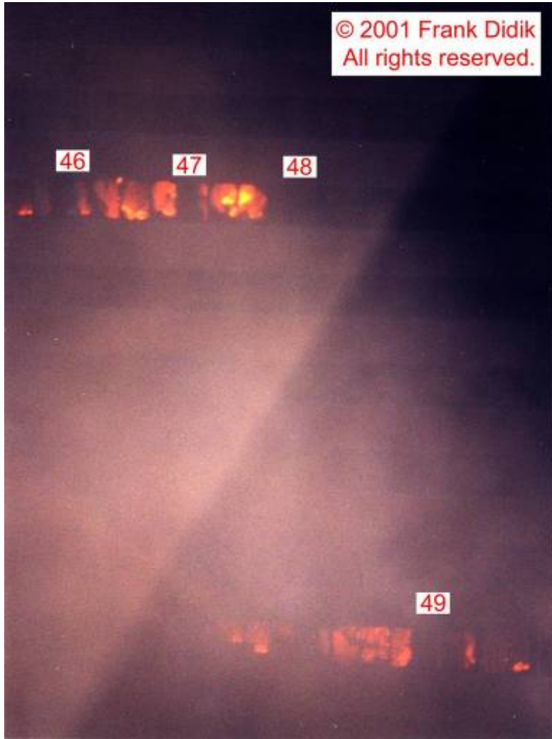
Figure 5–125. Cropped close-up photograph of the north face of WTC 7 taken within a few minutes of the image in Figure 5–124.
