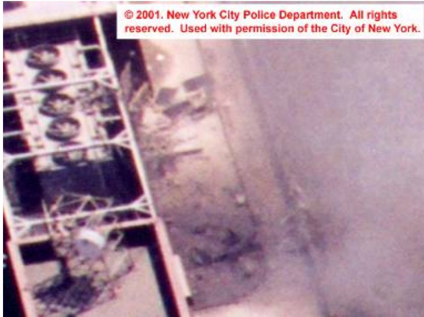
Figure 5–75. Cropped photograph, taken from a helicopter, showing the roof of WTC 7 from just north of due west.
