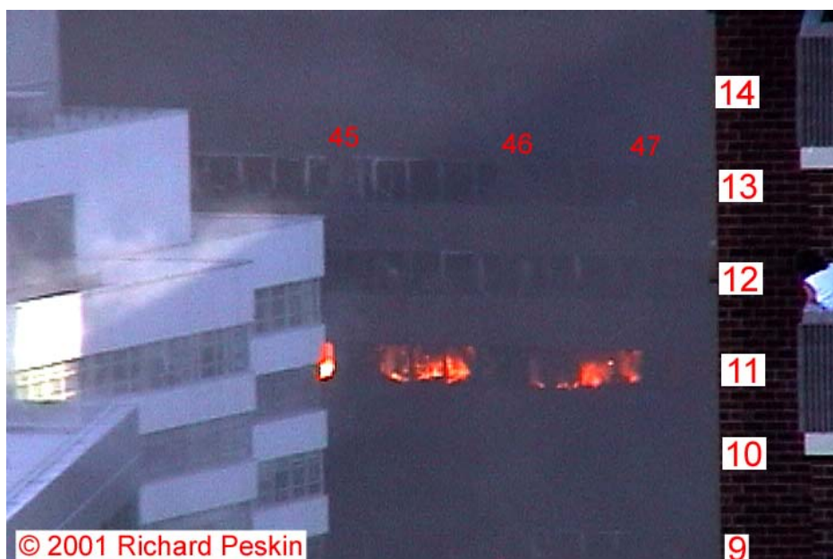
Figure 5–149. Frame from a video clip showing a close up view of the north face of WTC 7 at 4:38:14 p.m. ± 1 s. The video was shot from the same location as the frame in Figure 5–147. The image intensities were adjusted, and column and floor number have been added.
