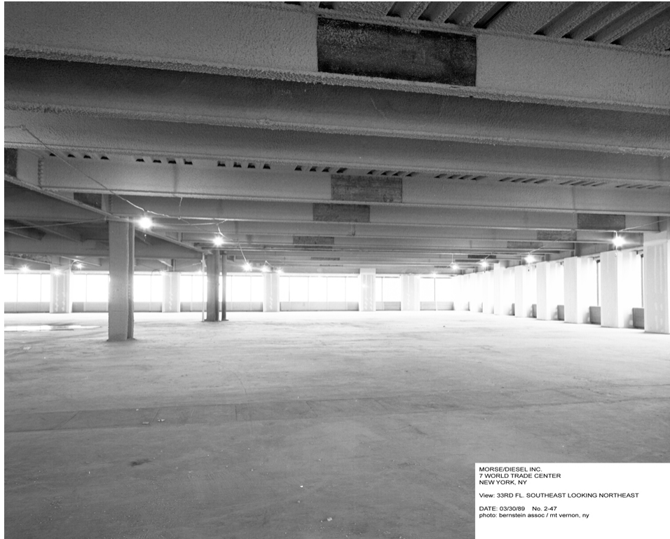
Figure 2–28. Photograph of Floor 33 during renovations showing SFRM on steel beams and metal deck, dated 03/30/89.
