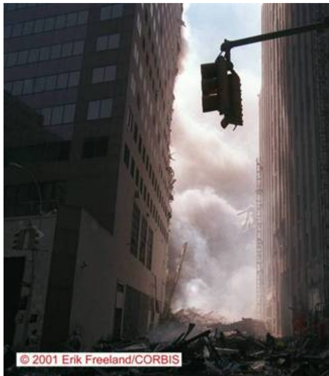
Figure 5–87. Cropped photograph of a partial view of the west face of WTC 7 looking down Washington Street between WTC 7 on the left and the Verizon Building on the right.
