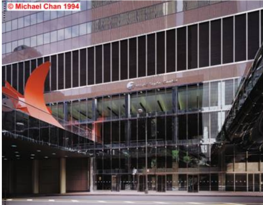
Figure 7–4. Photograph of the 3 rd floor exits from the south face of WTC 7. The Promenade is on the left and the enclosed pedestrian bridge is on the right.
