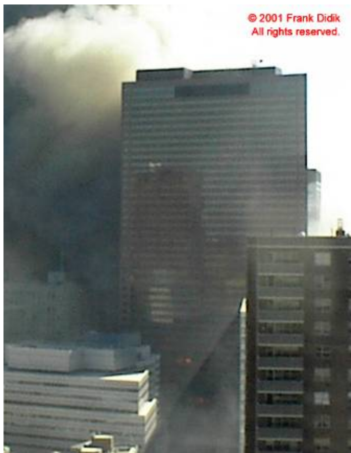
Figure 5–124. Cropped photograph of the north face of WTC 7 taken from a building located to the northwest looking down Greenwich Street at 3:10:46 p.m. ± 3 s. The intensities were adjusted.
