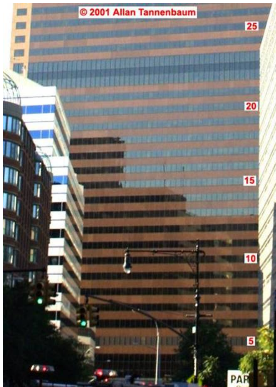
Figure 5–11. Enlargement of a portion of Figure 5–10 showing the lower floors of WTC 7. Floor numbers have been added, and the image has been enhanced.
