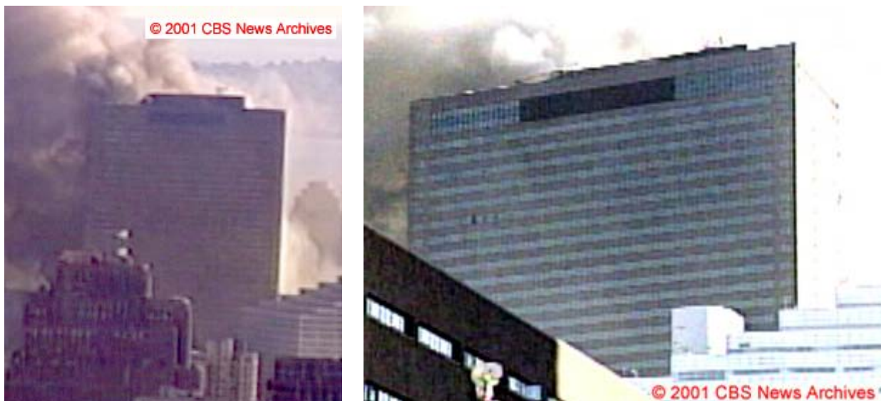
Figure 5–196. Cropped frames from the Camera 2 video clip and the Camera 3 video clip, showing the north face of WTC 7 2.0 \text{ s} \pm 0.1 \text{ s} after the east penthouse began to move downward.
