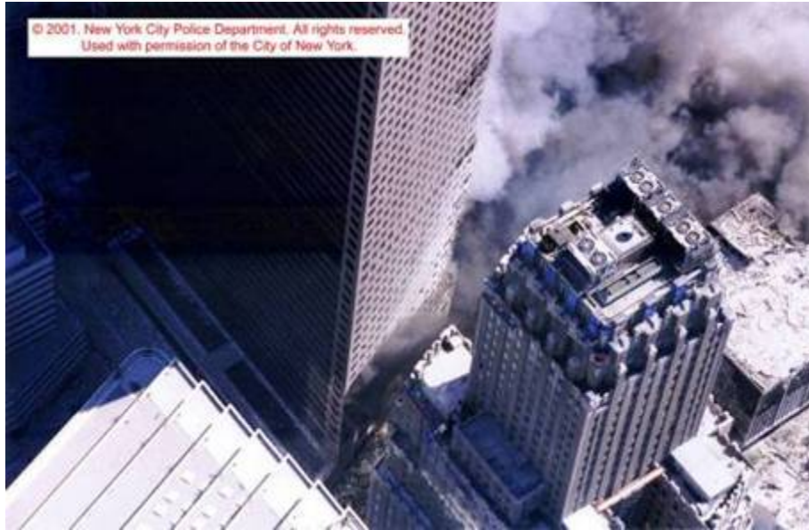
Figure 5–64. Photograph showing the north and west faces of WTC 7, shot from a helicopter between 2:15 p.m. and 2:45 p.m.
