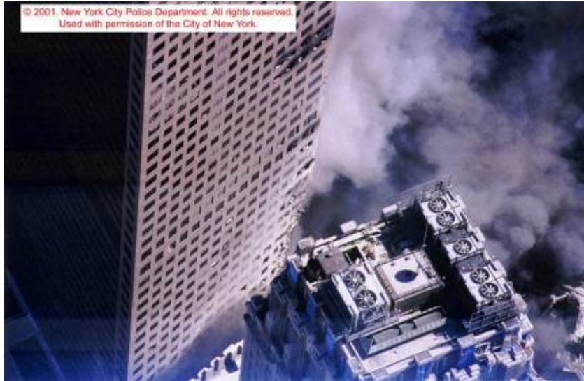
Figure 5–67. Photograph showing the north and west faces of WTC 7, shot from a helicopter between 2:30 p.m. and 3:00 p.m.
