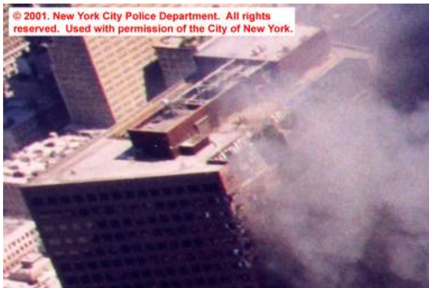
Figure 5–76. Cropped photograph showing the upper portion of WTC 7 as viewed from the southwest.
