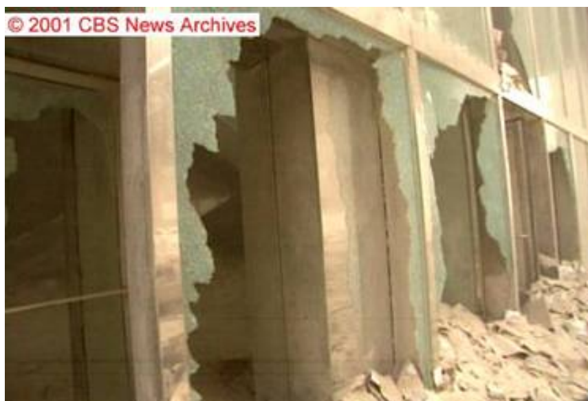
Figure 5–37. Video frame showing the ground floor of the south face of WTC 7, taken around 10:15 a.m. The column visible near the center is the base of column 25. The intensity levels have been enhanced.
