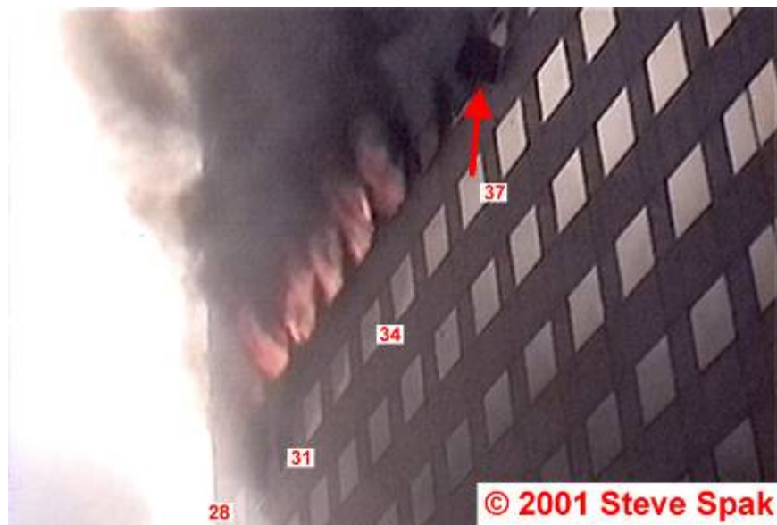
Figure 5–116. Frame from a video showing a portion of the east face of WTC 7 between 2:15 p.m. and 2:27 p.m.
