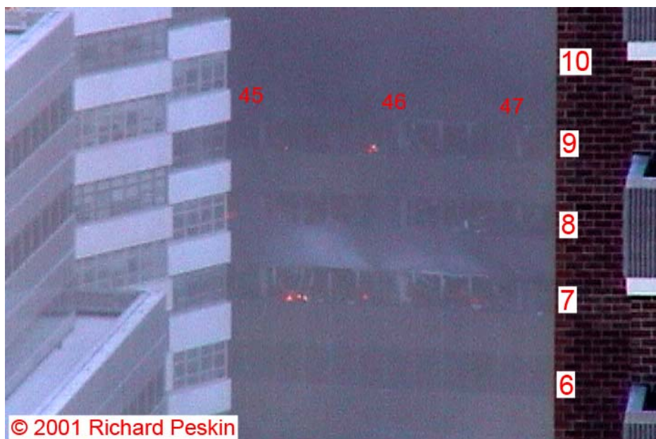
Figure 5–148. Frame from a video clip showing a close up view of the north face of WTC 7 at 4:38:11 p.m. ± 1 s. The video was shot from the same location as the frame in Figure 5–147. The image intensities were adjusted, and column and floor number have been added.
