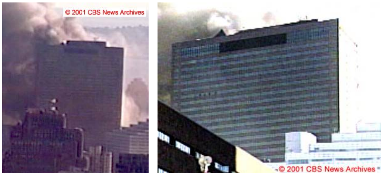
Figure 5–195. Cropped frames from the Camera 2 video clip and the Camera 3 video clip, showing the north face of WTC 7 1.7 \text{ s} \pm 0.1 \text{ s} after the east penthouse began to move downward.
