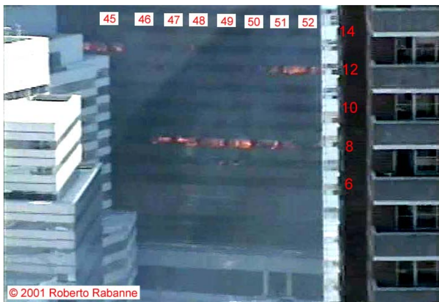
Figure 5–131. This frame from a video shot from a building to the northwest of WTC 7 was taken around 3:50:13 p.m. with an uncertainty of \pm 3 min. The intensities have been adjusted and column and floor numbers added.
