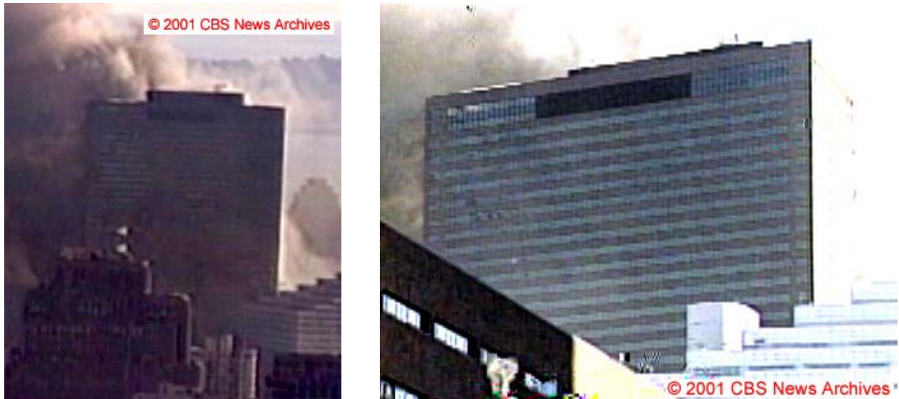
Figure 5-197. Cropped frames from the Camera 2 video clip and the Camera 3 video clip, showing the north face of WTC 7 3.5 \text{ s} \pm 0.1 \text{ s} after the east penthouse began to move downward.
