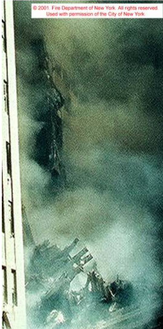
Figure 5–57. Expanded portion of Figure 5–56 showing damage on the south face of WTC 7. The contrast of the image has been enhanced.
