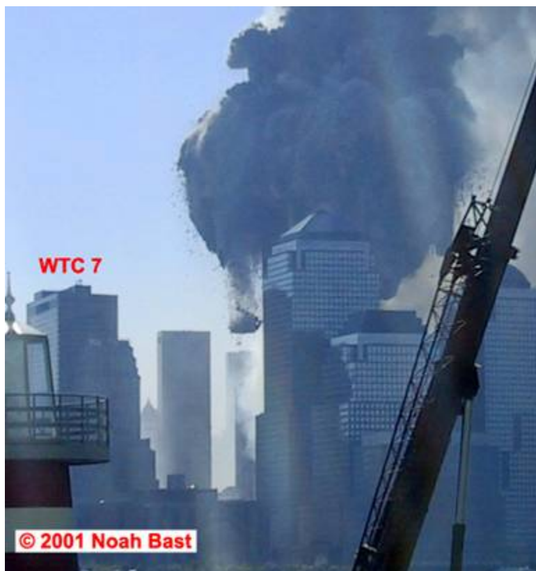
Figure 5–43. Cropped photograph showing the collapse of WTC 1, taken from just north of west of the WTC site 7.3 s ± 0.2 s after initiation of the collapse.
