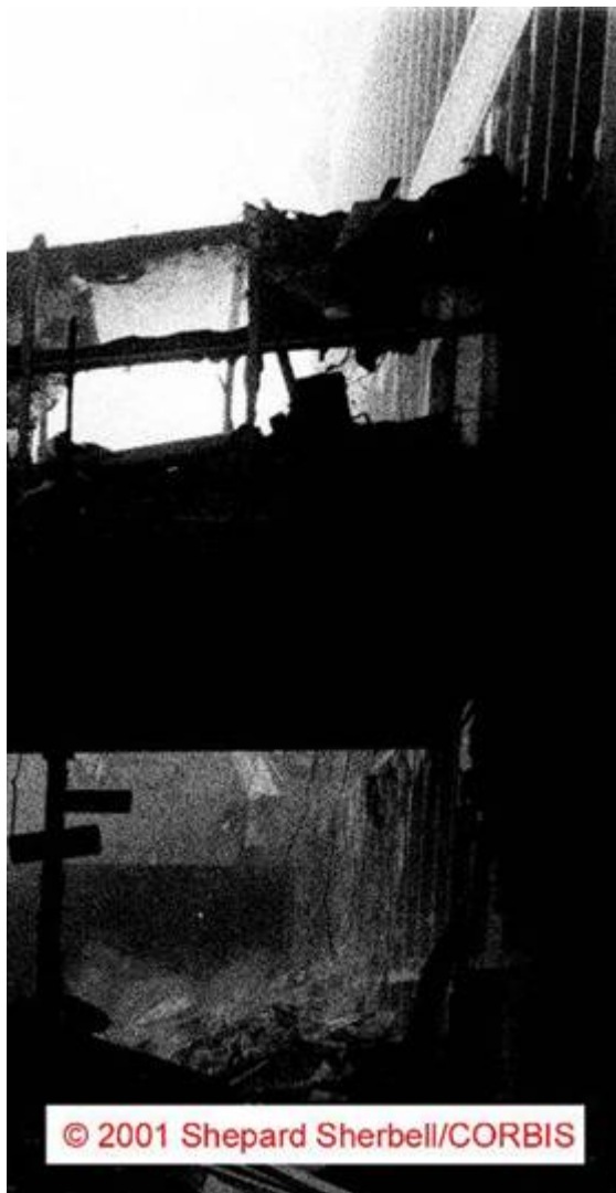
Figure 5–71. Enlargement of the photograph in Figure 5–70 showing the south face of WTC 7.
