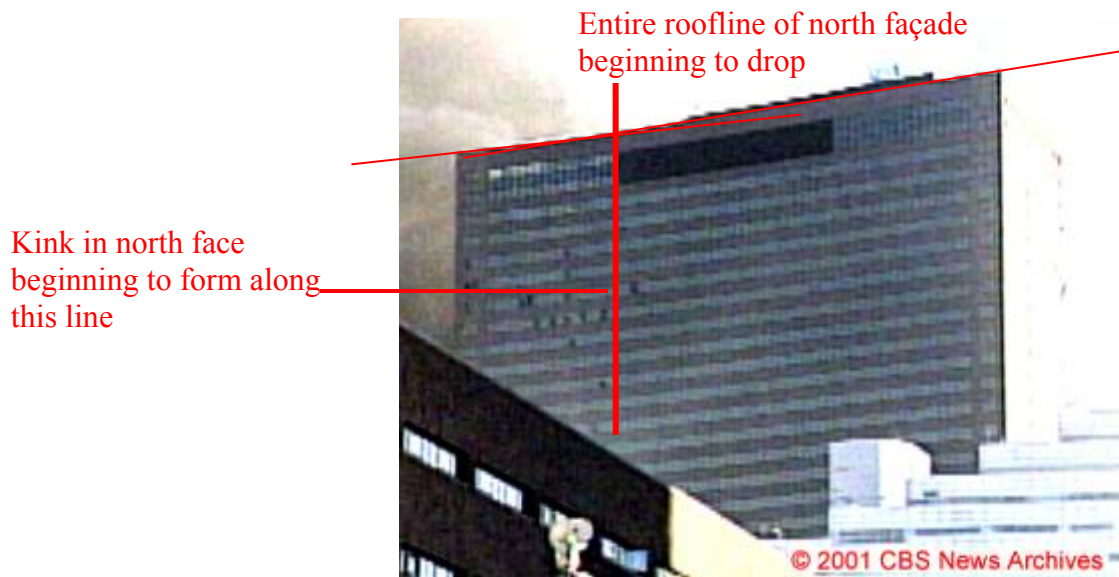
Figure 8–5. Global collapse of WTC 7 begins about seven seconds after the onset of collapse of the east penthouse.
