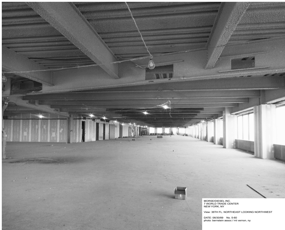
Figure 2–29. Photograph of Floor 36 during renovations, showing SFRM on steel beams and metal deck, looking dated 06/30/89.
