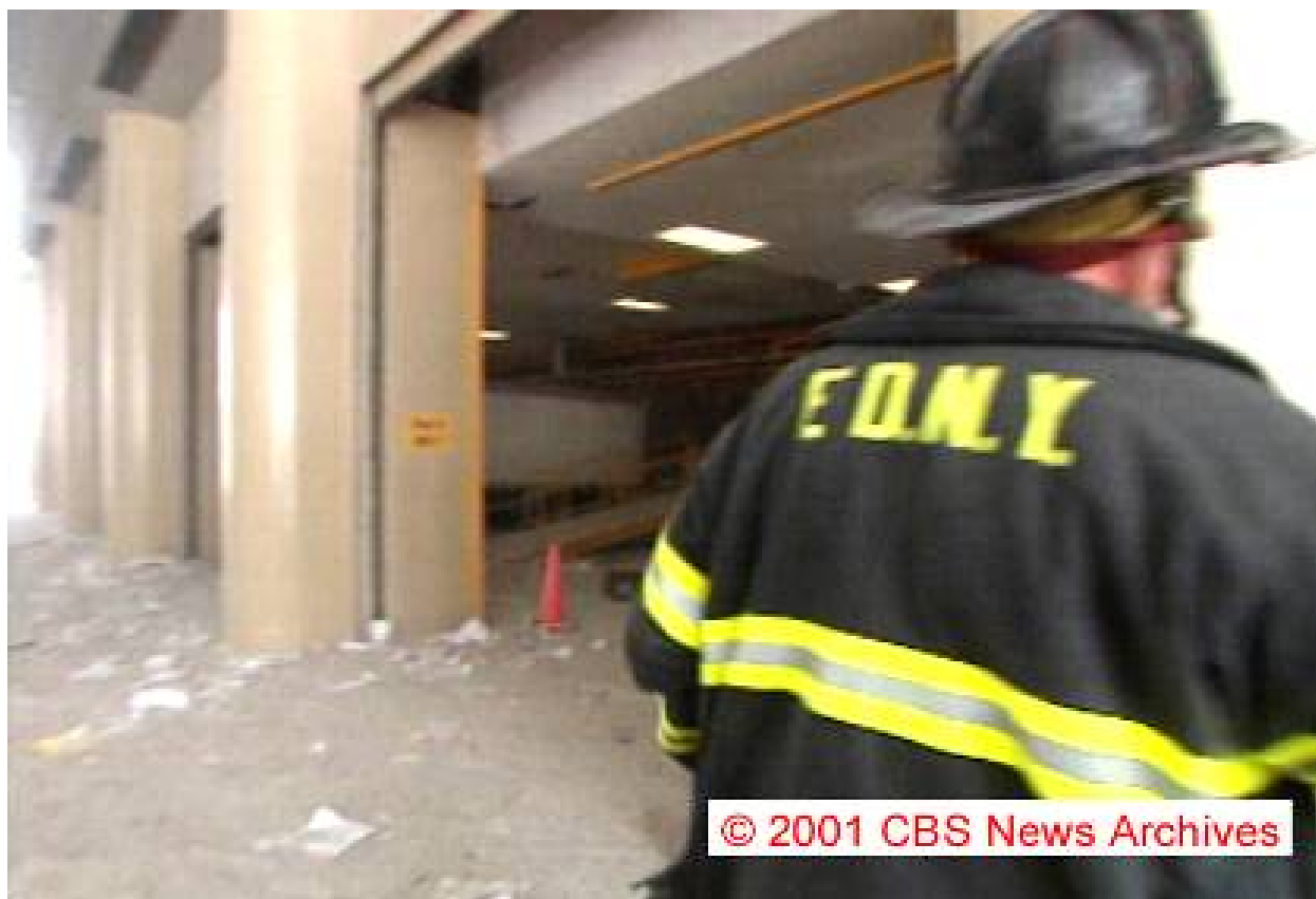
Figure 5–17. Frame from a video showing one of the doorways located below the Promenade that led to the WTC 7 loading dock located on the 1 st and 2 nd floors. The image has been enhanced.
