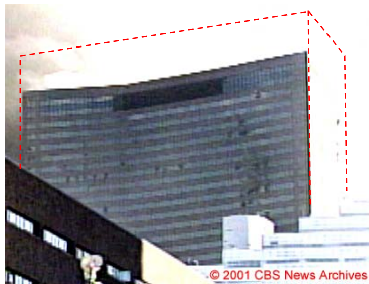
Figure 8–6. Entire building continues to collapse.
