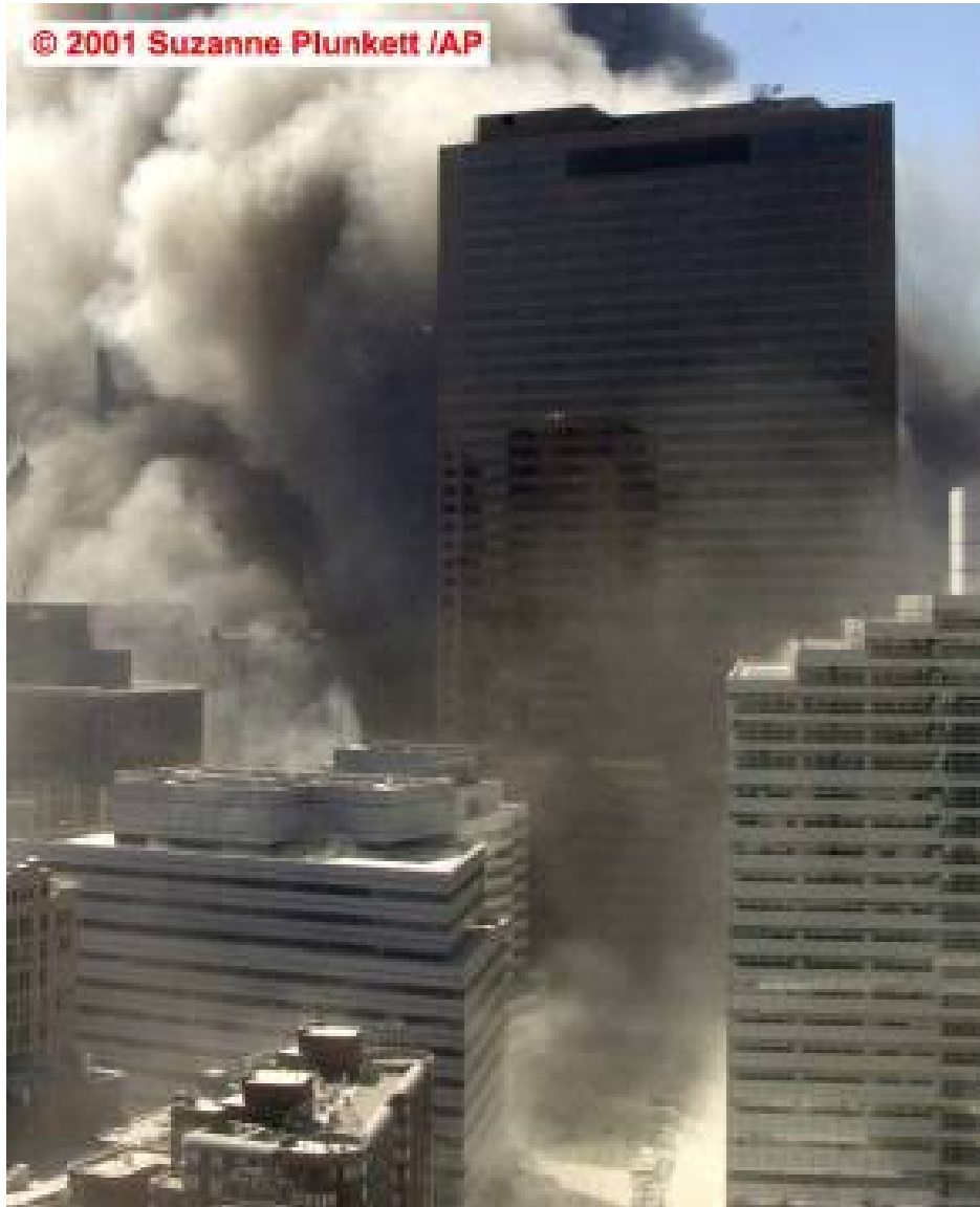
Figure 5–104. Cropped photograph showing the north face of WTC 7, shot at 11:28:15 a.m. from the upper story of a nearby building looking down Greenwich. The intensity levels have been adjusted.
