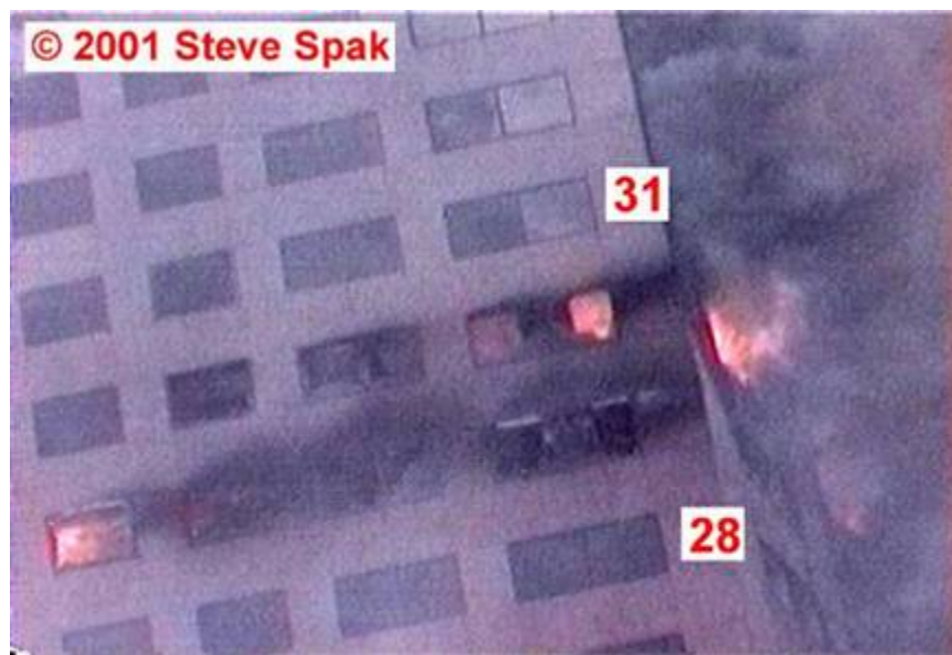
Figure 5–111. Frame from a video clip showing fires near the southwest corner of WTC 7 on the 29 th and 30 th floors around 12:28 a.m. ± 3 min.
