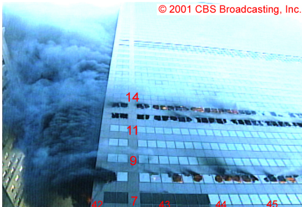
Figure 5–141. Frame from a video shot from near the corner of West Broadway and Barclay Street showing the eastern side of the north face of WTC 7 between 3:53 p.m. and 4:02 p.m.
