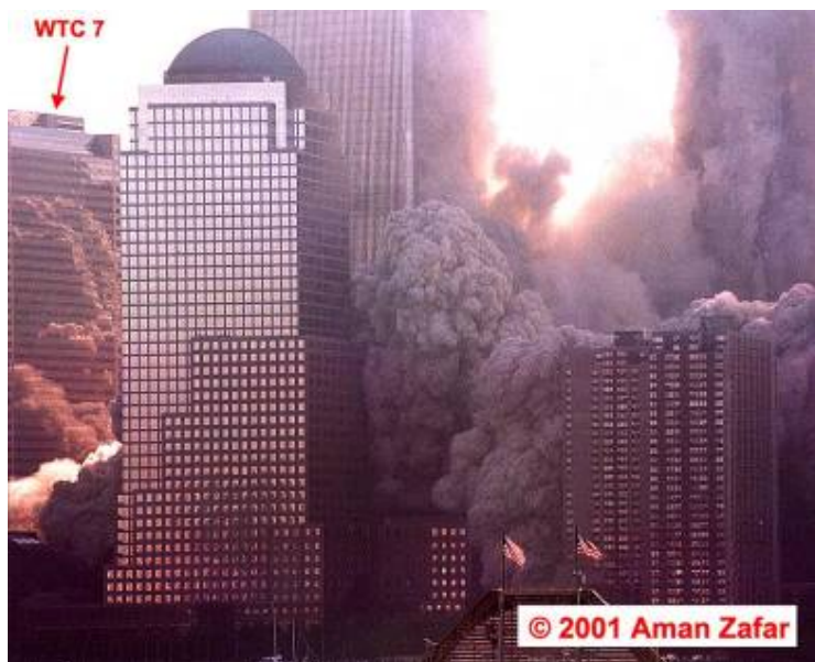
Figure 5–34. Photograph of the collapse of WTC 2 taken at 9:59:15 a.m. (with an uncertainty of 5 s). An arrow has been added to identify WTC 7. The original image has been cropped and the intensities have been adjusted.
