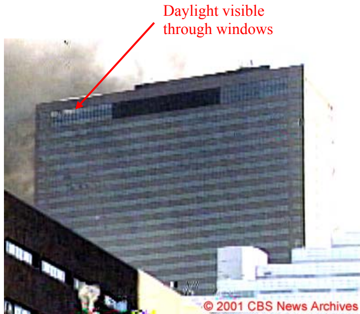
Figure 8–4. Daylight visible where roof collapsed on east side of building.
