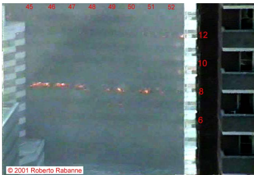
Figure 5–139. This frame from a video shot from a building to the northwest of WTC 7 was taken around 3:54:14 p.m. with an uncertainty of \pm 3.5 min. The intensities have been adjusted and column and floor numbers added.
