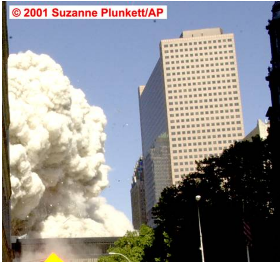
Figure 5–35. Cropped photograph showing the dust cloud from the collapse of WTC 2 approaching the south face of WTC 7, taken from just east of the corner of Fulton Street and Broadway at 9:59:24 a.m. (estimated uncertainty of 5 s). The intensity levels have been adjusted.
