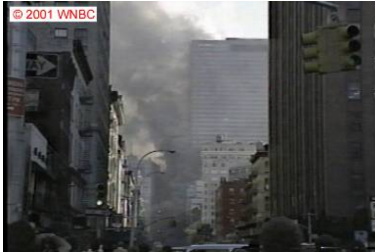
Figure 5–187. Earliest frame from the Camera 4 video, showing the north face of WTC 7.
