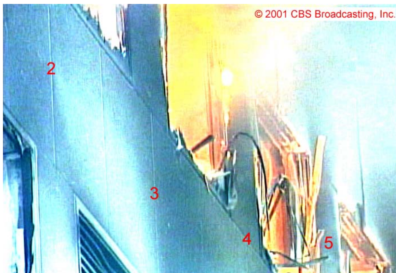
Figure 5–133. View of the west face of WTC 7 taken from a video recorded from inside the lobby of 123 Barclay Street around 3:41:30 ± 5 min.
