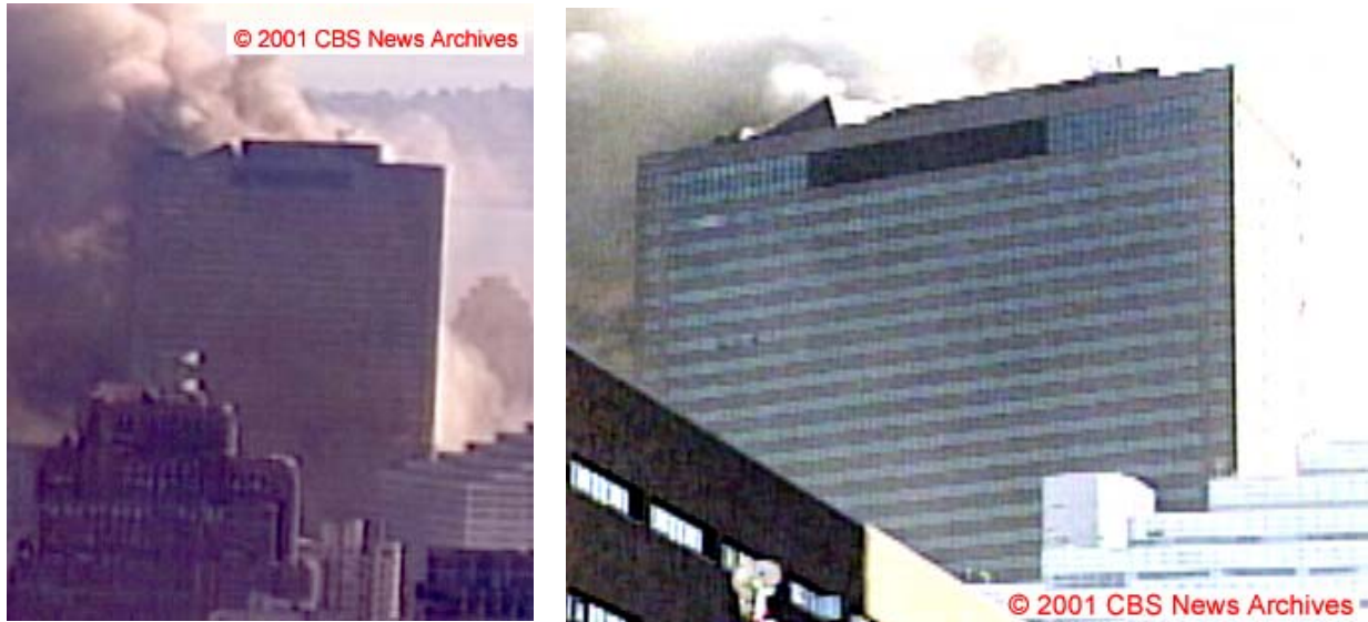
Figure 5–194. Cropped frames from the Camera 2 video clip and the Camera 3 video clip, showing the north face of WTC 7 1.3 \text{ s} \pm 0.1 \text{ s} after the east penthouse began to move downward. The intensities have been adjusted.
