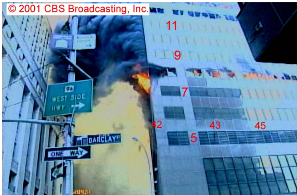
Figure 5–142. Frame taken from a video shot near the corner of West Broadway and Barclay Street showing the lower northeast corner of WTC 7 between 3:55 p.m. and 4:04 p.m.
