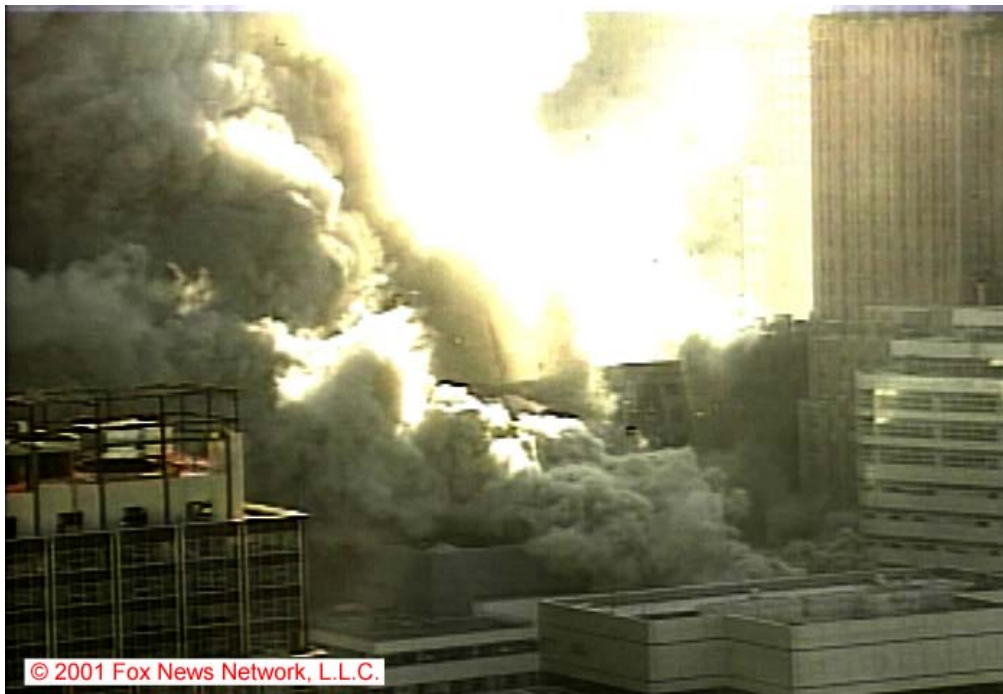
Figure 5-216. Frame from the Camera 6 video clip in Figure 5-189, showing the north face of WTC 7 13.0 \text{ s} \pm 0.2 \text{ s} after the east penthouse began to move downward. The intensities have been adjusted.
