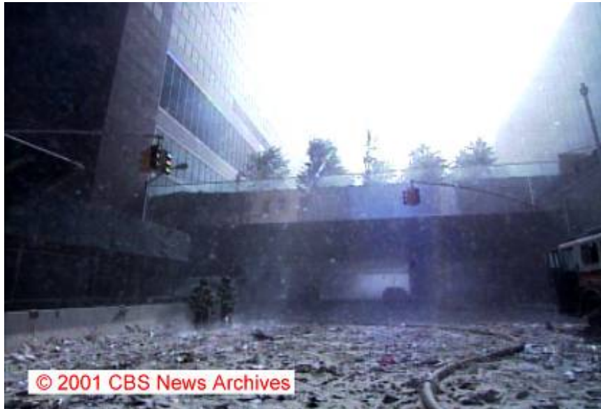
Figure 5–18. An image from a video, shot from Vesey Street and looking toward the east, shows the south face of WTC 7 and the Promenade crossing over to WTC 6. The video was recorded around 10:15 a.m. on September 11. The intensity levels of the image have been adjusted.
