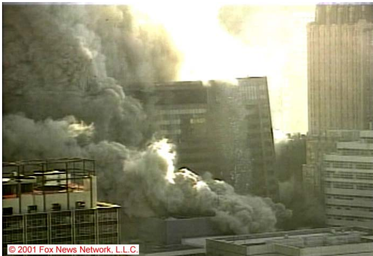
Figure 5–214. Frame from the Camera 6 video clip in Figure 5–189, showing the north face of WTC 7 12.0 s \pm 0.2 s after the east penthouse began to move downward. The intensities have been adjusted.
