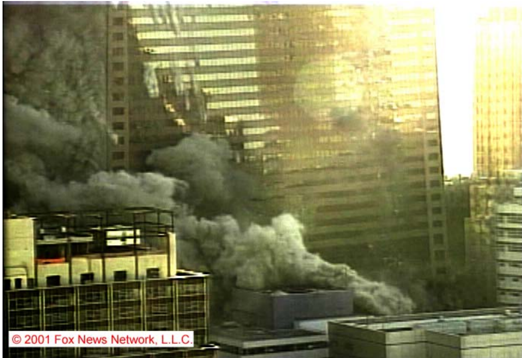
Figure 5–209. Frame from the Camera 6 video clip in Figure 5–189, showing the north face of WTC 7 10.0 \text{ s} \pm 0.2 \text{ s} after the east penthouse began to descend. The intensities have been adjusted.
