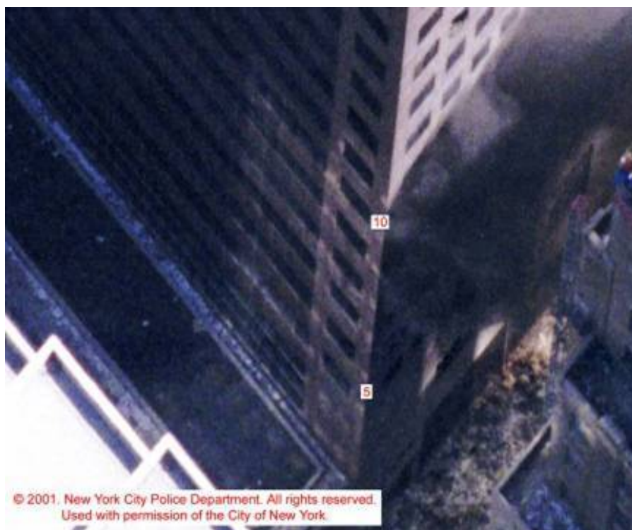
Figure 5–113. Enlargement of a portion of the photograph shown in Figure 5–64 emphasizing areas on the lower floors of WTC 7 near the northwest corner.
