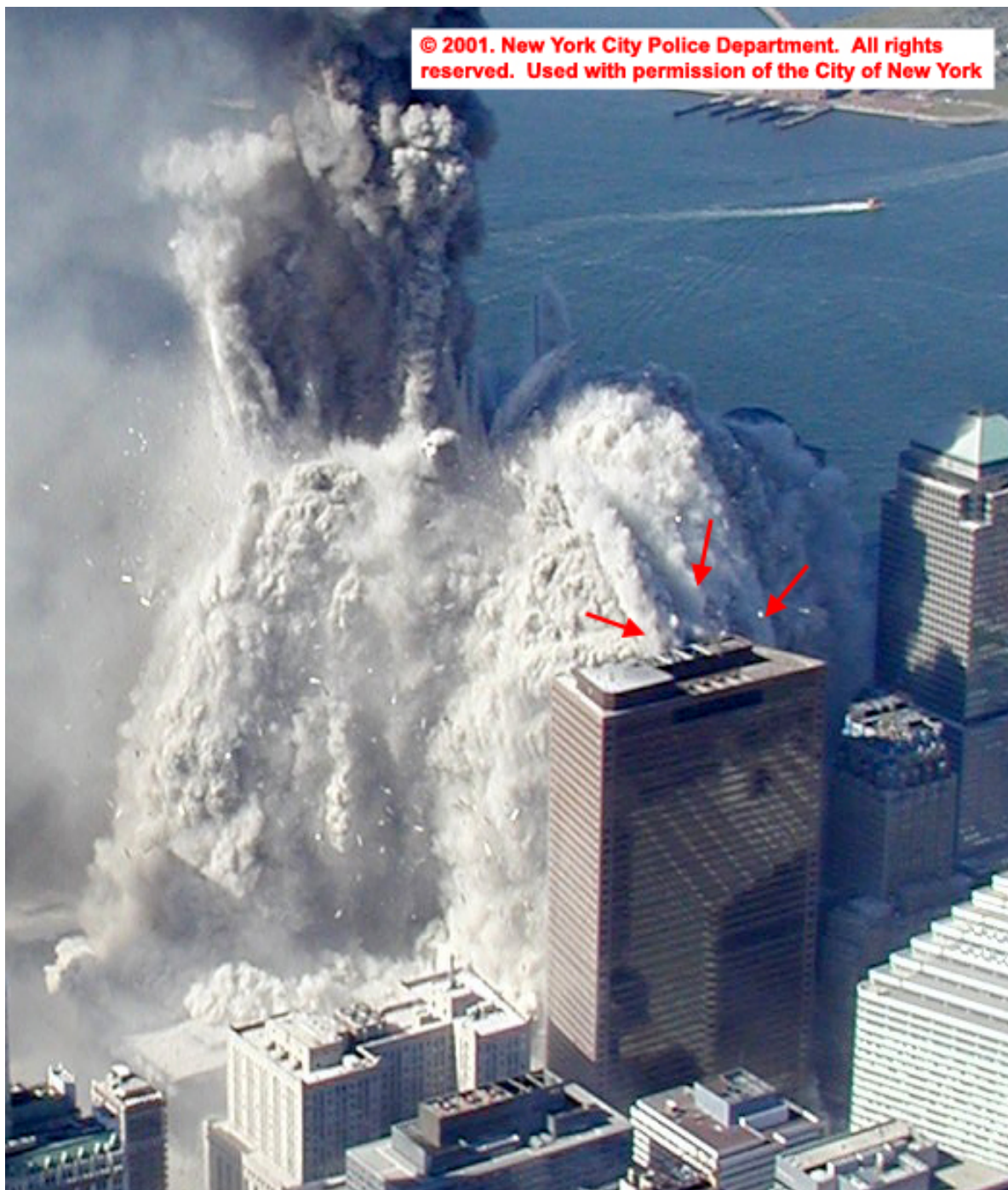
Figure 5–42. Aerial photograph shot 14 s \pm 0.5 s after WTC 1 began to collapse. Arrows mark arcs formed by debris that seemed to be ejected outwards from the debris cloud.
