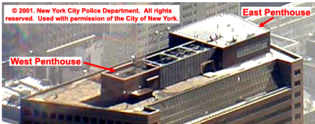
Figure 5–8. Photograph taken from the southwest at 10:22:50 a.m. on September 11 showing the mechanical systems and penthouses on the roof of WTC 7.
