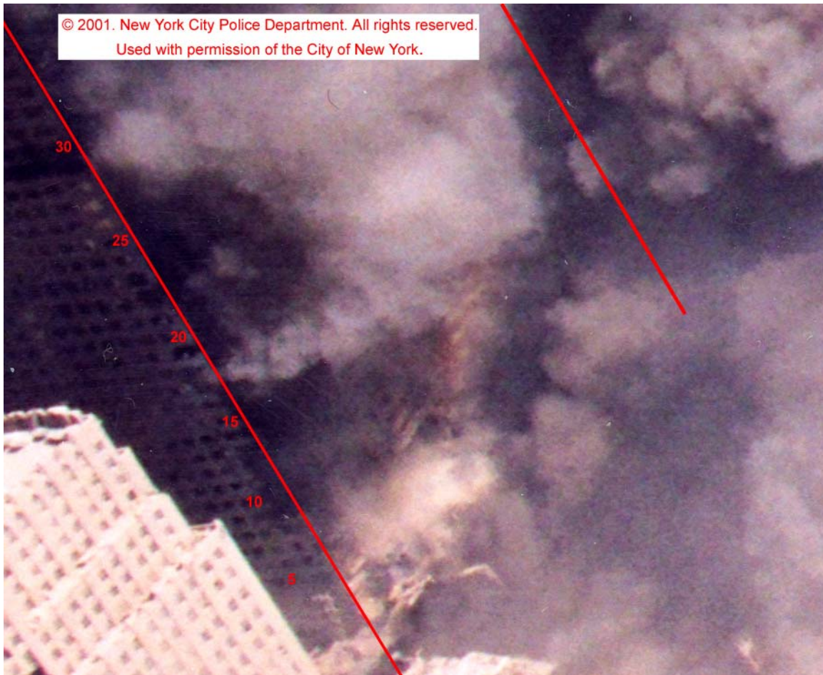
Figure 5–61. Enlarged portion of Figure 5–60 showing the south face of WTC 7. The section has been enhanced by adjusting the intensity levels. The red lines indicate the west and east edges. Floor numbers have been added.
