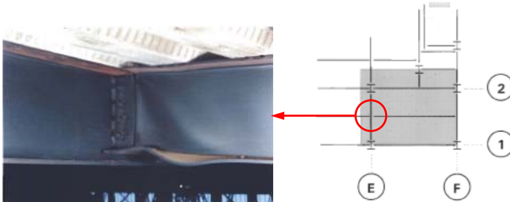
Figure 8–17. Floor beam buckling at symmetrical framing to girder.
