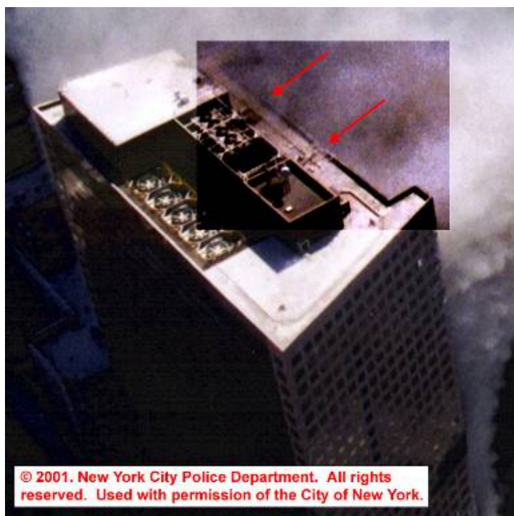
Figure 5–74. Cropped photograph, taken from a helicopter, showing the roof of WTC 7 from the northwest.
