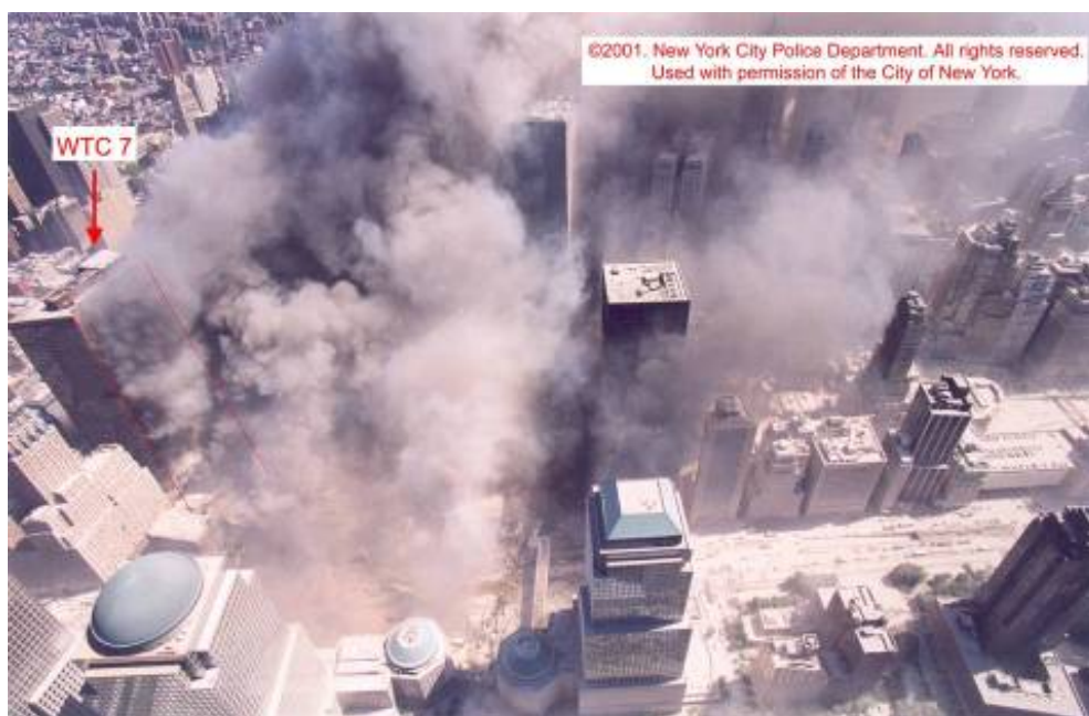
Figure 5–60. Photograph of the WTC site shot around 12:35 p.m. from a helicopter. The red lines identify the west and east edges of the south face of WTC 7.
