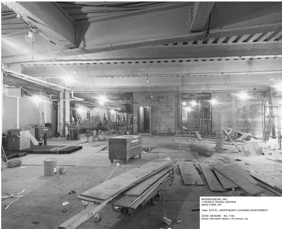
Figure 2–27. Photograph of Floor 5 during renovations showing SFRM on steel beams and metal deck, dated 08/30/89.
