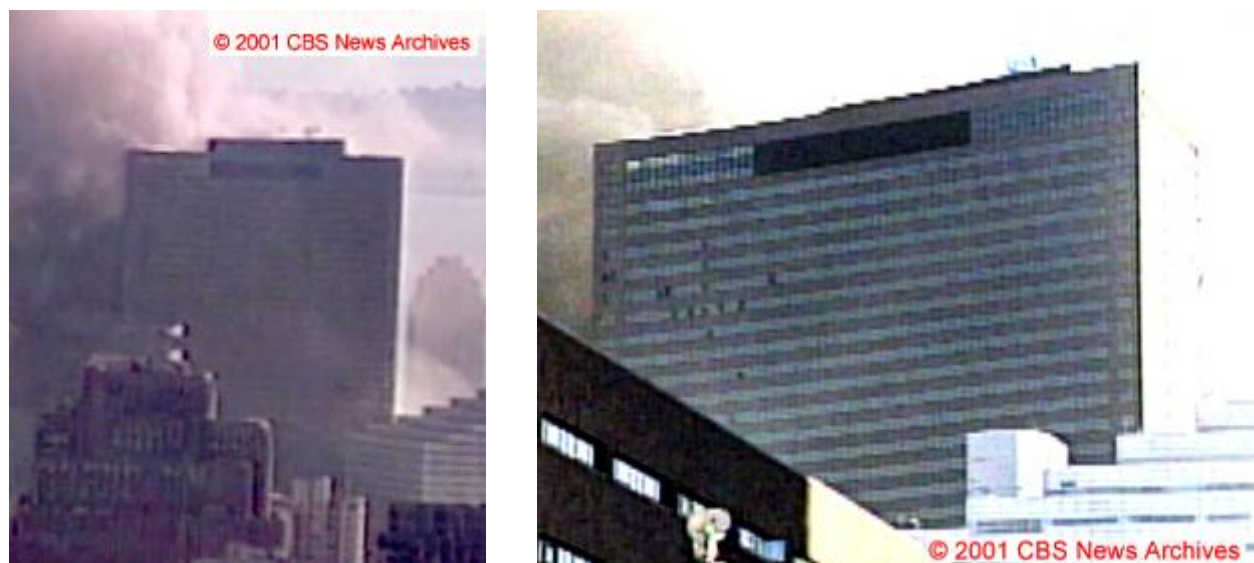
Figure 5–200. Cropped frames from the Camera 2 video clip in Figure 5–185 and the Camera 3 video clip in Figure 5–186, showing the north face of WTC 7 7.5 s \pm 0.1 s after the east penthouse began to move downward.
