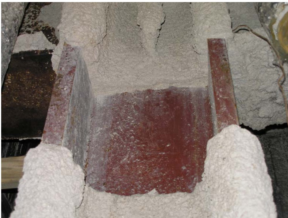
Figure 2–35. Column with removed SFRM and intact primer.
