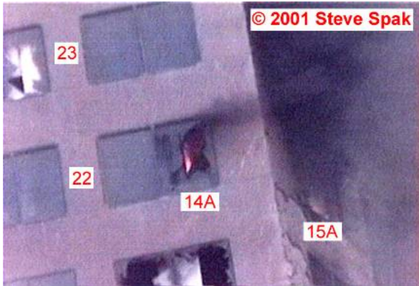
Figure 5-109. Frame from a video clip showing the southwest corner of WTC 7 around the 22 nd floor.
