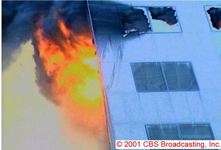
Figure 5-143. Frame from a video shot near the corner of West Broadway and Barclay Street showing a close up of the northeast corner of WTC 7 at the 8 th floor between 3:56 p.m. and 4:05 p.m.
