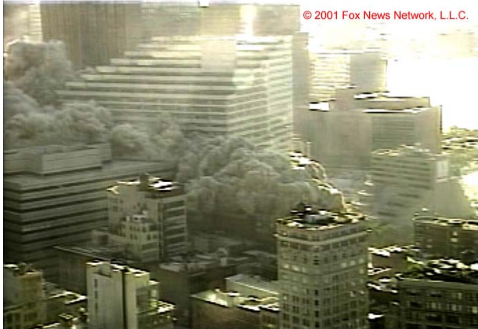
Figure 5–217. Frame from the Camera 6 video clip in Figure 5–189, showing the dust-laden flow generated by the collapse of WTC 7, 22.0\text{ s} \pm 0.2\text{ s} after the east penthouse began to move downward. The intensities have been adjusted.
