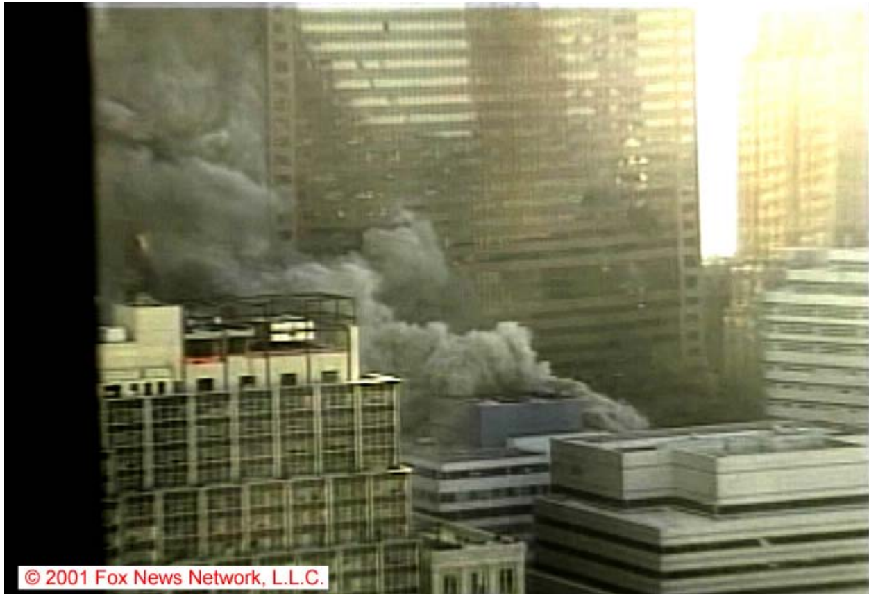
Figure 5–207. Frame from the Camera 6 video clip in Figure 5–189, showing the north face of WTC 7 9.0 \text{ s} \pm 0.2 \text{ s} after the east penthouse began to move downward.
