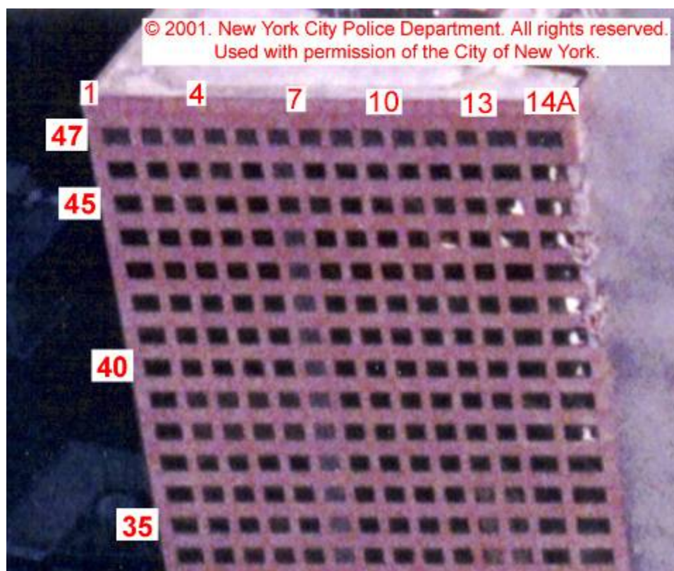
Figure 5–84. Cropped photograph showing the west face of WTC 7, taken from a helicopter around 3:00 p.m. The intensity levels have been adjusted.
