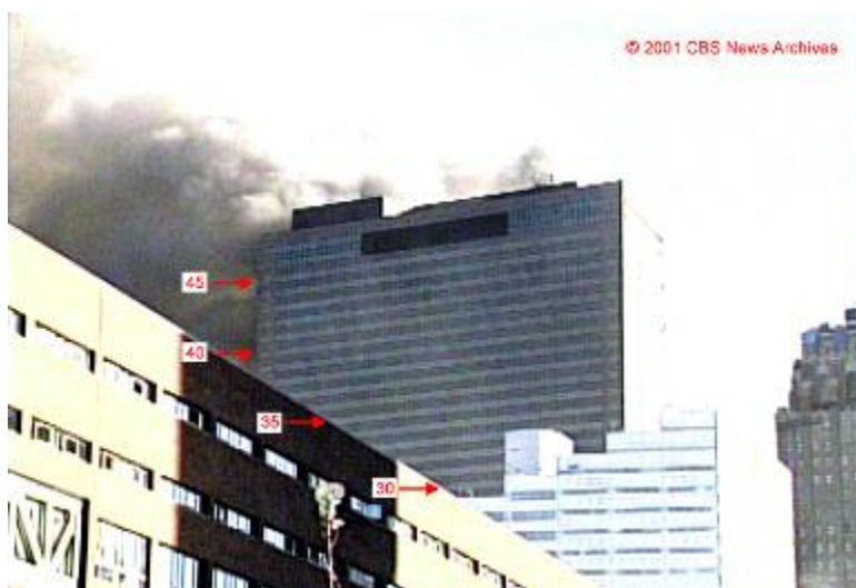
Figure 5–186. Frame from the Camera 3 video showing the north face of WTC 7 (in center) seconds before the east penthouse began to fall into the building.
