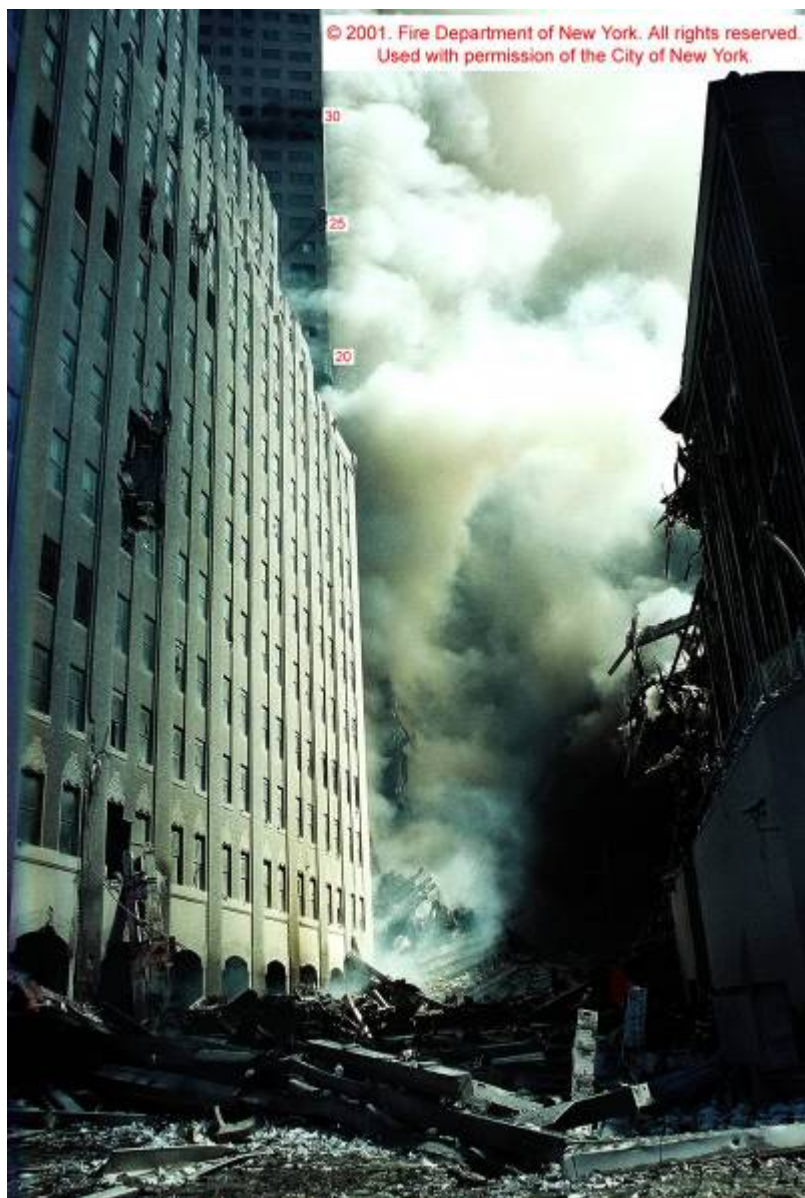
Figure 5–56. Photograph of damage on the south face of WTC 7, shot looking down Vesey Street between the Verizon Building (left) and WTC 6 (right), shortly after 1:30 p.m. The intensity levels have been adjusted.
