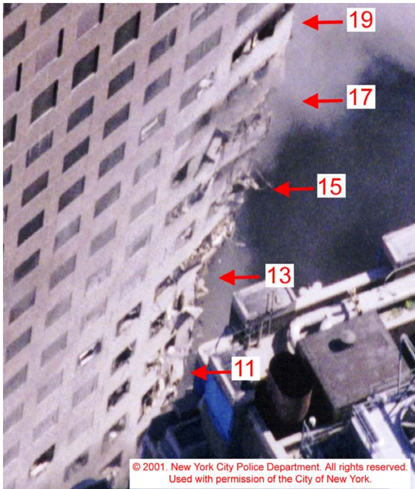
Figure 5–68. Enlargement of an area from the photograph in Figure 5–67 showing part of the west face of WTC 7.
