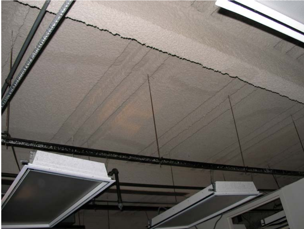
Figure 2–34. Floor beams with intact SFRM.
