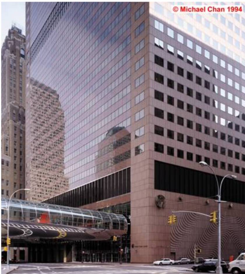
Figure 5–16. Photograph showing the lower southeast corner of WTC 7.
