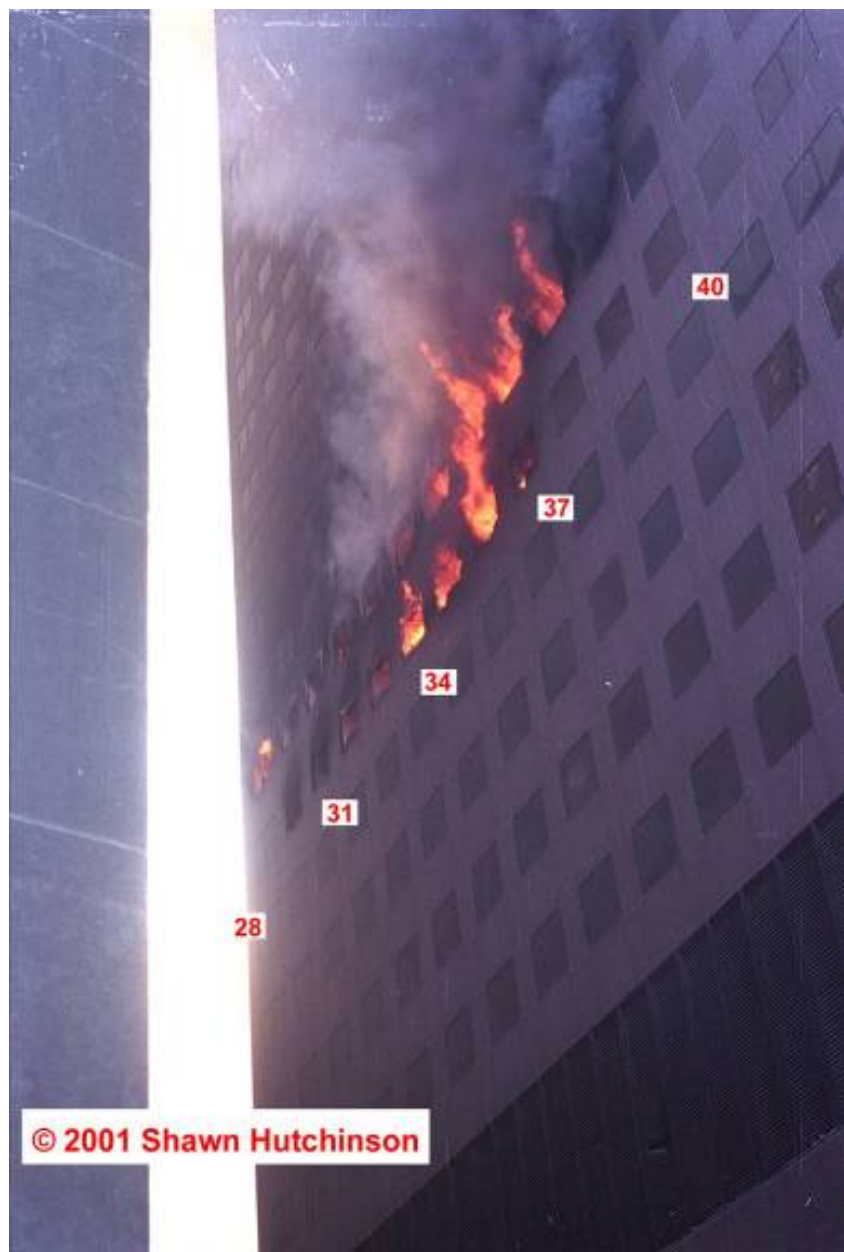
Figure 5–118. Photograph of the east face of WTC 7 taken at some time after 2:28:43 p.m. from near the corner of West Broadway and Barclay Street.
