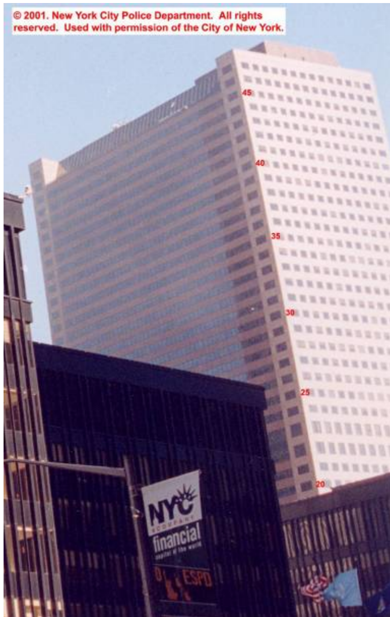
Figure 5–14. Photograph showing upper portions of the south and east faces of WTC 7, taken from near the corner of Church Street and Liberty Street on September 11 at 9:51:45 a.m. The two buildings in the foreground are WTC 4 (left) and WTC 5 (right). Floor numbers have been added, and the image was cropped and enhanced.
