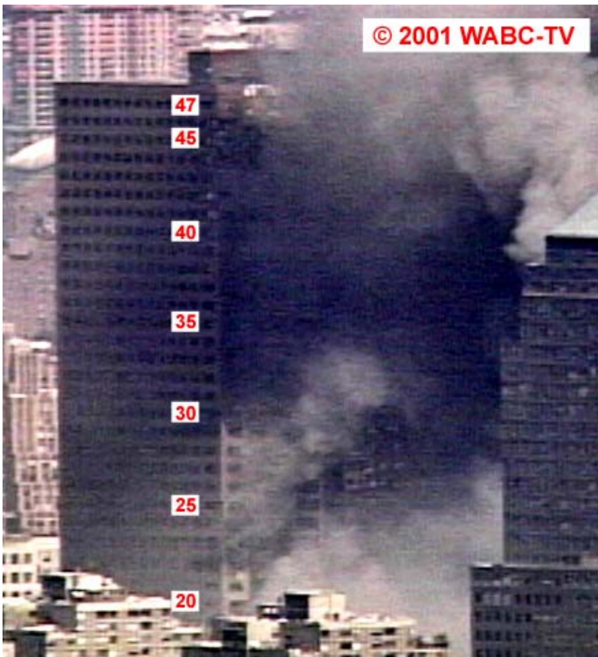
Figure 5–82. Cropped view of the south face of WTC 7 taken from a video shot from a helicopter hovering to the southwest of the WTC site around 1:00 p.m. The intensity levels have been adjusted.
