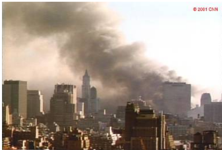
Figure 5–184. Frame from the Camera 1 video, showing the north face of WTC 7 (on right) seconds before the east penthouse began to fall into the building.
