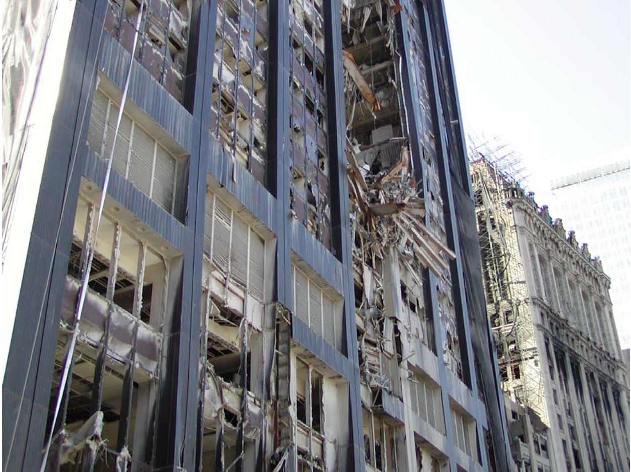
Figure 2–30. Exterior view of damage to the north face of 130 Liberty Street by debris falling from WTC 2.
