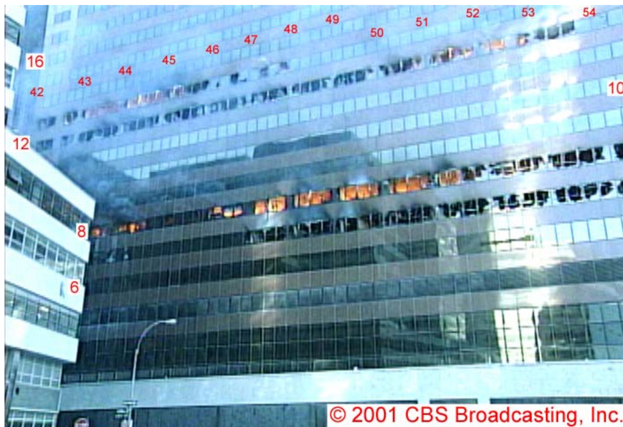
Figure 5–136. Frame taken from a video shot from near the corner of Greenwich Street and Park Place showing the north face of WTC 7 between 3:49 p.m. and 3:54 p.m. The building on the left is 30 West Broadway. The intensities have been adjusted, and column and floor numbers have been added.
