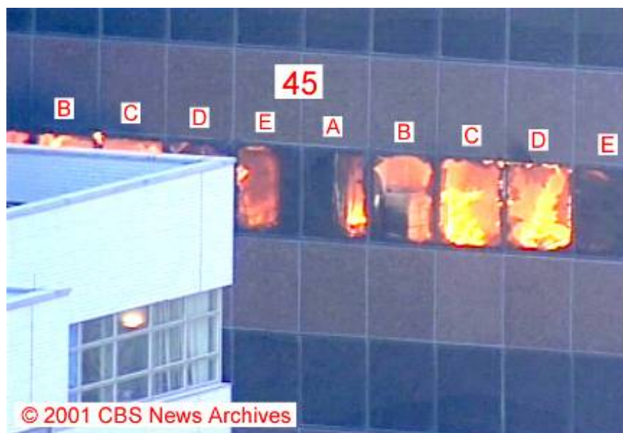
Figure 5–122. Frame taken from a video clip shot looking down on WTC 7 from a building to the northwest shows the fires along a length of the north side of the 12 th floor of WTC 7.
