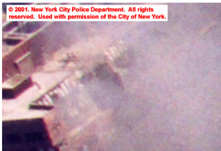
Figure 5–77. Enlargement of the area of damage on the roof and south sides of the 46 th and 47 th floors of WTC 7 in Figure 5–76.
