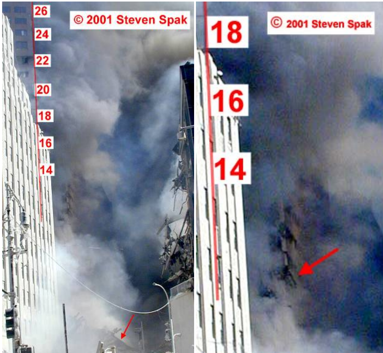
Figure 5–53. Two enlargements from Figure 5–52, showing the south face of WTC 7. The vertical red line indicates the location of the southwest corner of the building. Floor number locations were determined as described in the text. The red arrow in the left enlargement identifies debris that may be from the Promenade, and the arrow on the right indicates a characteristic damage pattern.
