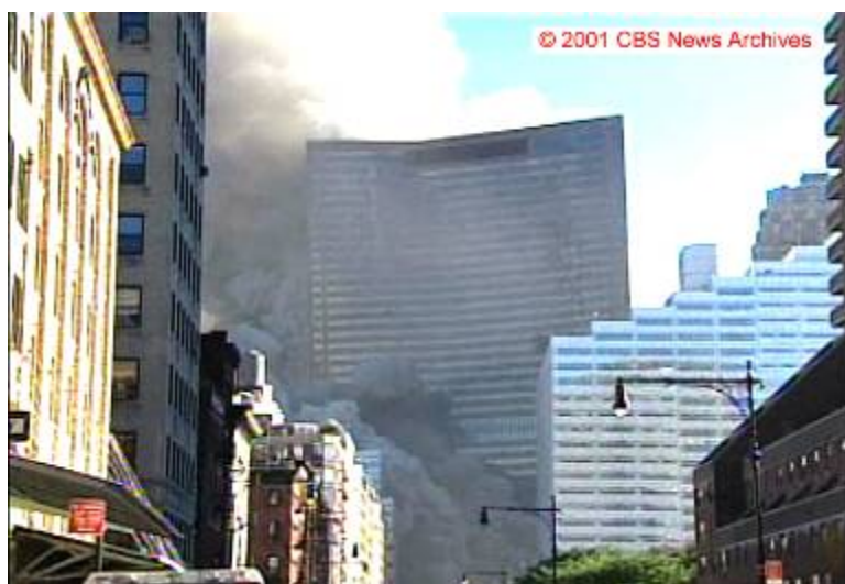
Figure 5-192. Earliest frame from the Camera 9 video, showing the north face of WTC 7.
