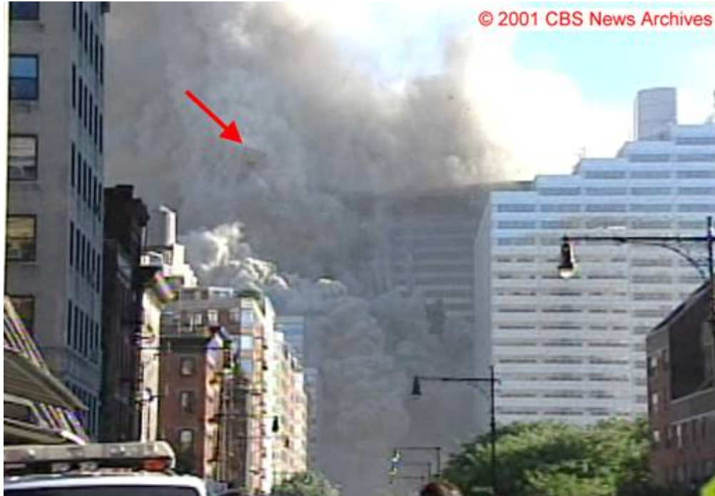
Figure 5-215. Frame from the Camera 9 video clip in Figure 5-192, showing the north face of WTC 7 12.0 \text{ s} \pm 0.2 \text{ s} after the east penthouse began to move downward. The arrow indicates a section of the northeast corner of the building that has broken away from the main section of the building. The intensities have been adjusted.
