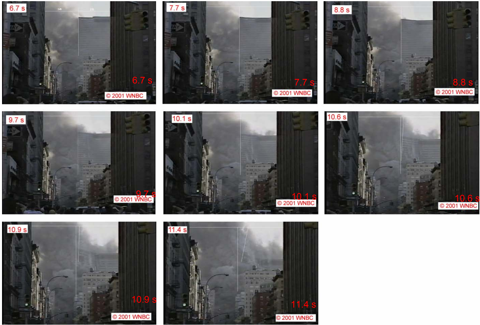
Figure 5–204. Images from the Camera 4 video clip showing relative movement of the northeast edge of WTC 7 during its global collapse.
