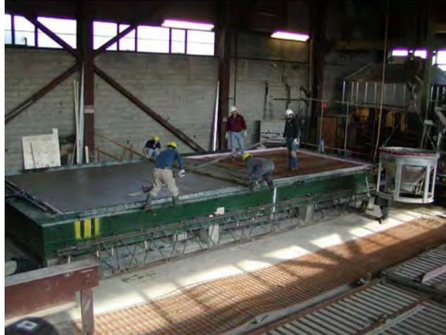
**Figure 2–22. Fabrication of 35 ft span ASTM E 119 test assembly.**
